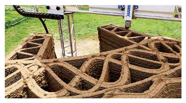
Figure 2.3.7. WASP is using its Crane 3D printer to build TECLA | Image via WASP (3dNatives, 2020).
