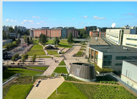
Figure 5.8 - Overview of the roof landscape
